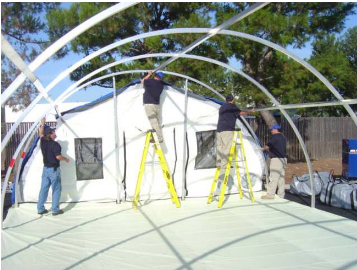
Setting up the a 25 bed tent facility
